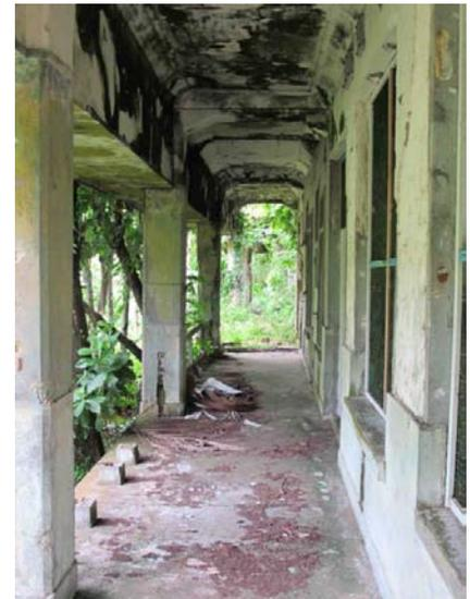
**Figure 5.12** Weakened concrete supports on the west end of the Japanese RDF Administration and Communications building contrast with the well-preserved and enclosed eastern portion of the structure.
