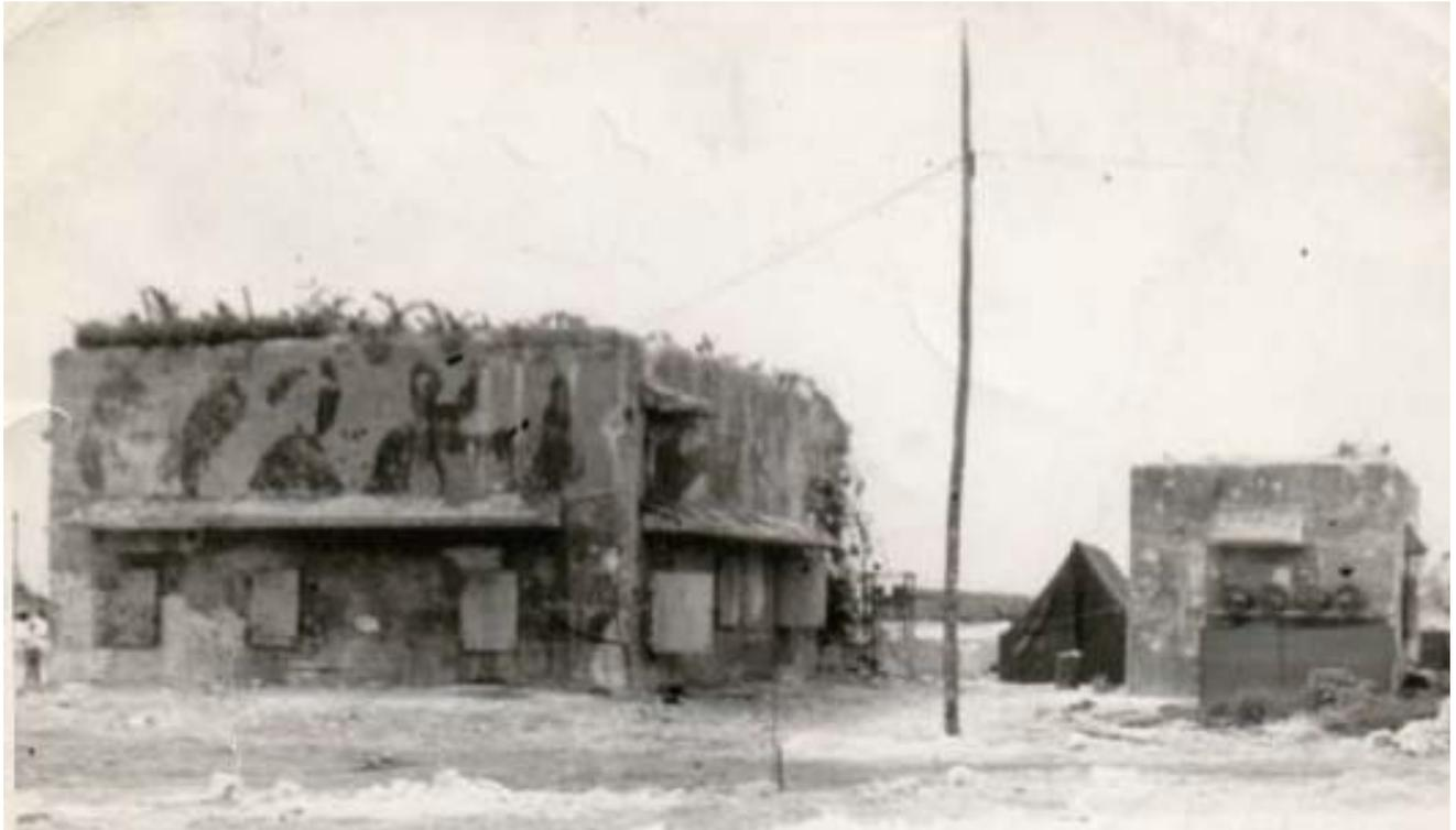
**Figure 5.44** Japanese main power plant (AB36) and concrete fuel storage building (AB37) in 1944. Note the camouflage paint and the plantings on the roof. (NARA:RG127)
