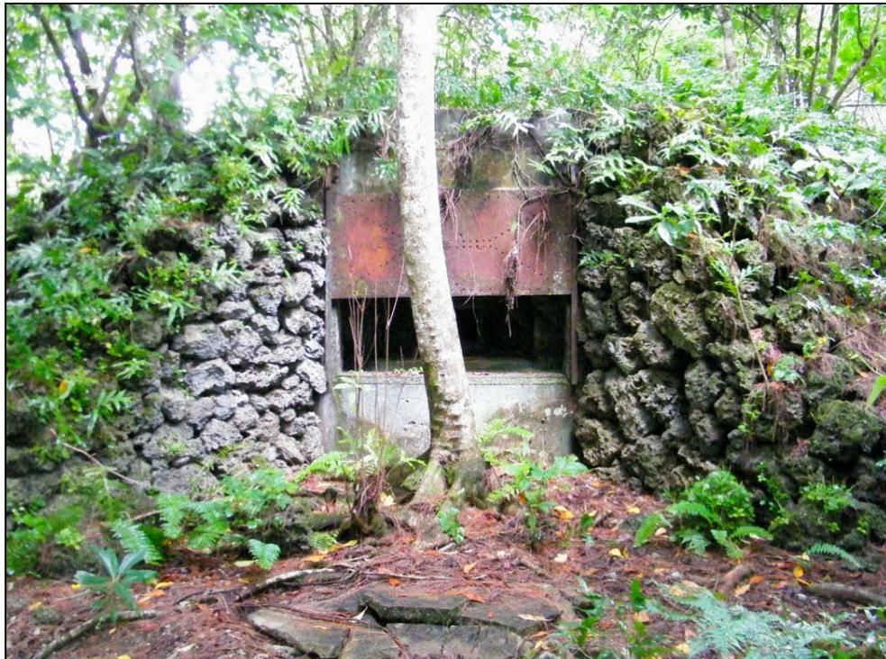
**Figure 4.35** Firing ports and sliding iron blast doors remained in good condition at AB142 in 2010.
