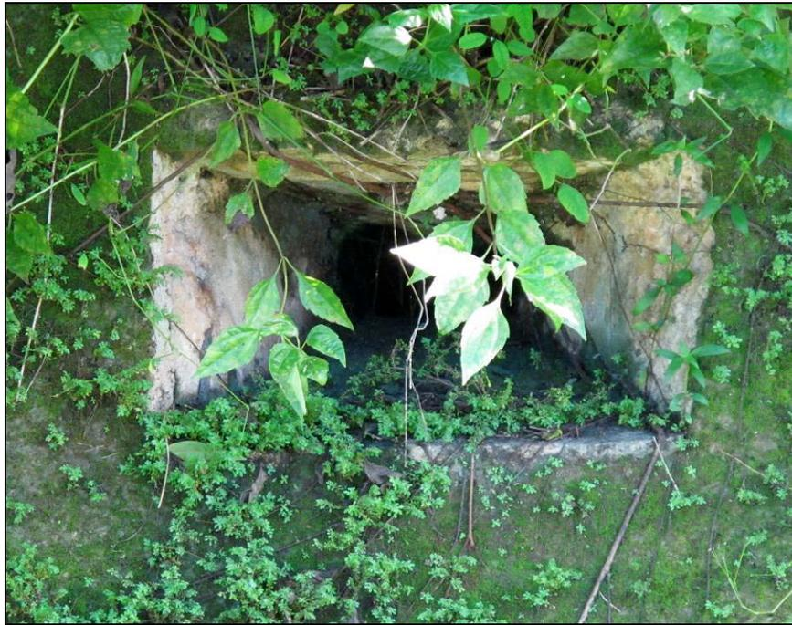
**Figure 8.5** One of the fire ports that were cut into the former phosphate loading platform.
