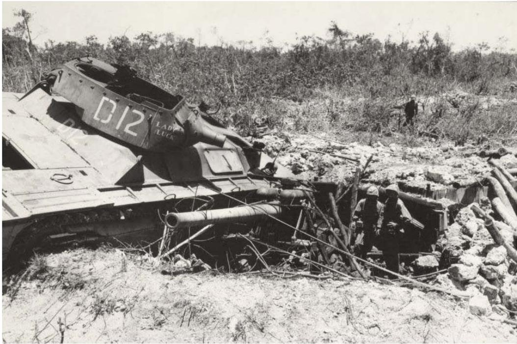
**Figure 4.25** The 'Lady Luck' LVT(A)4 in 1944, stuck after falling through the roof of AB187, a Japanese 120 mm gun position. (NARA; RG 127)
