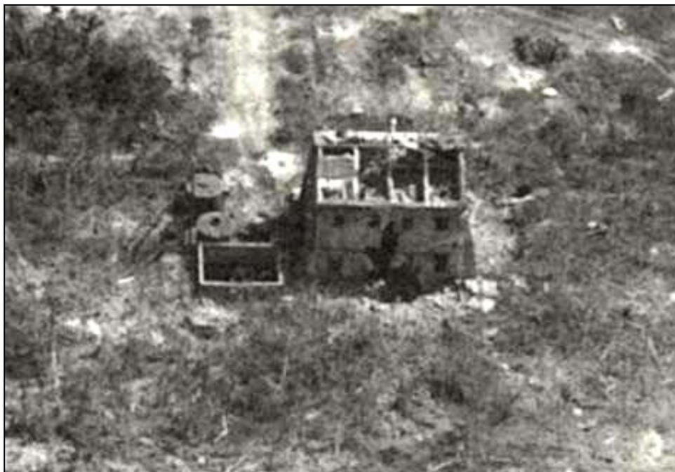
**Figure 5.38** Detail from figure 5.37. It appears that the second story floor of the building survived the assault but was lost later, probably as the wood decomposed.
