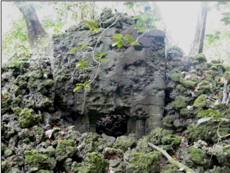
**Figure 3.24** Same view of AB60 in 2010, showing partial damage to coral revetment, probably from visitor traffic.
