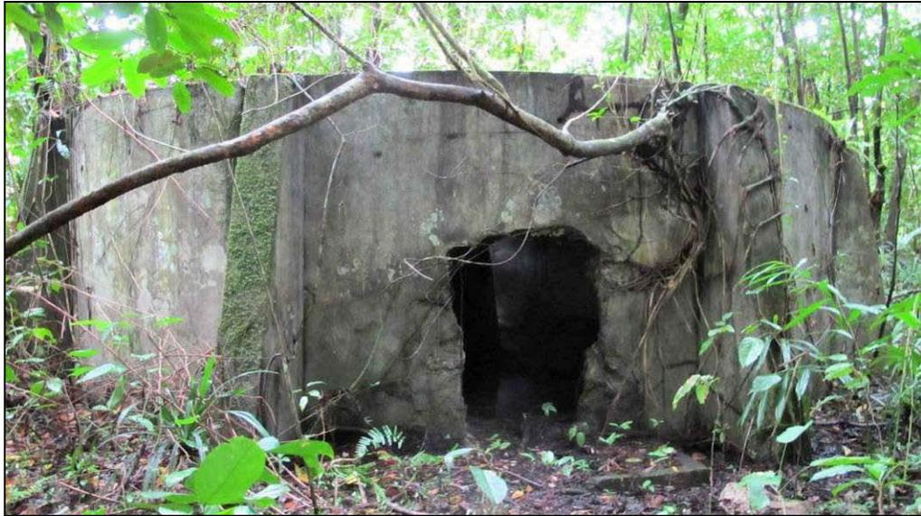
**Figure 5.34** AB24, one of two concrete water tanks that once served the bath house at AB22. Doorways may have installed to convert it into a defensive bunker.
