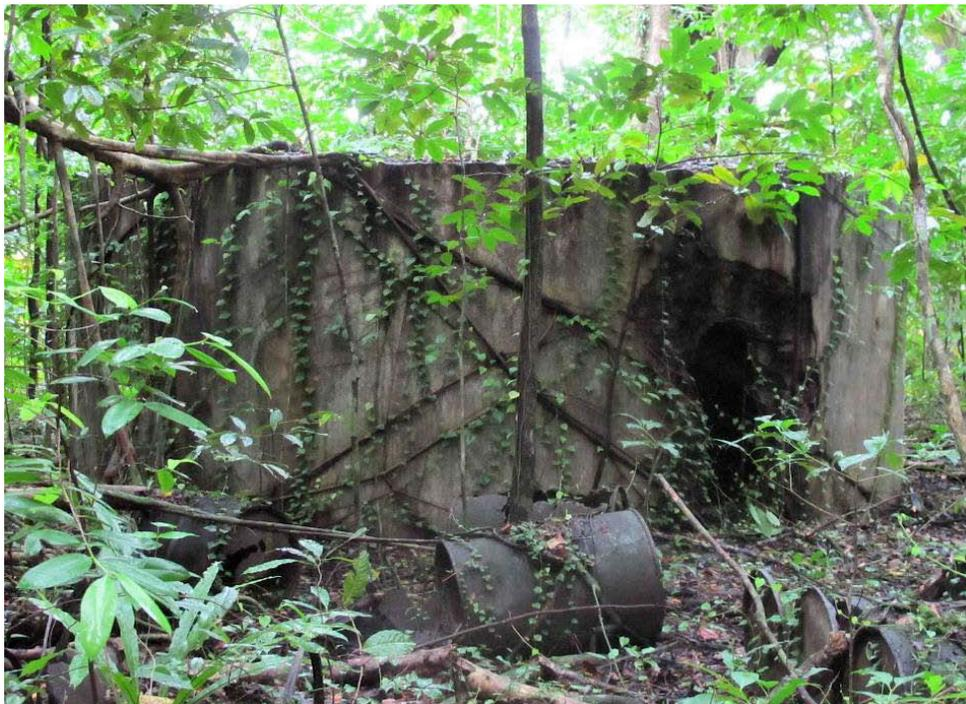
**Figure 5.33** AB23, a concrete Japanese water cistern has a doorway blasted through one side.
