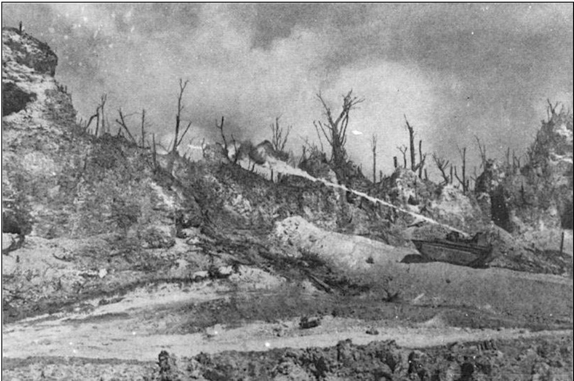
**Figure 7.34** Ramp in use by an AVT equipped with a flamethrower. (NARA; RG127)
