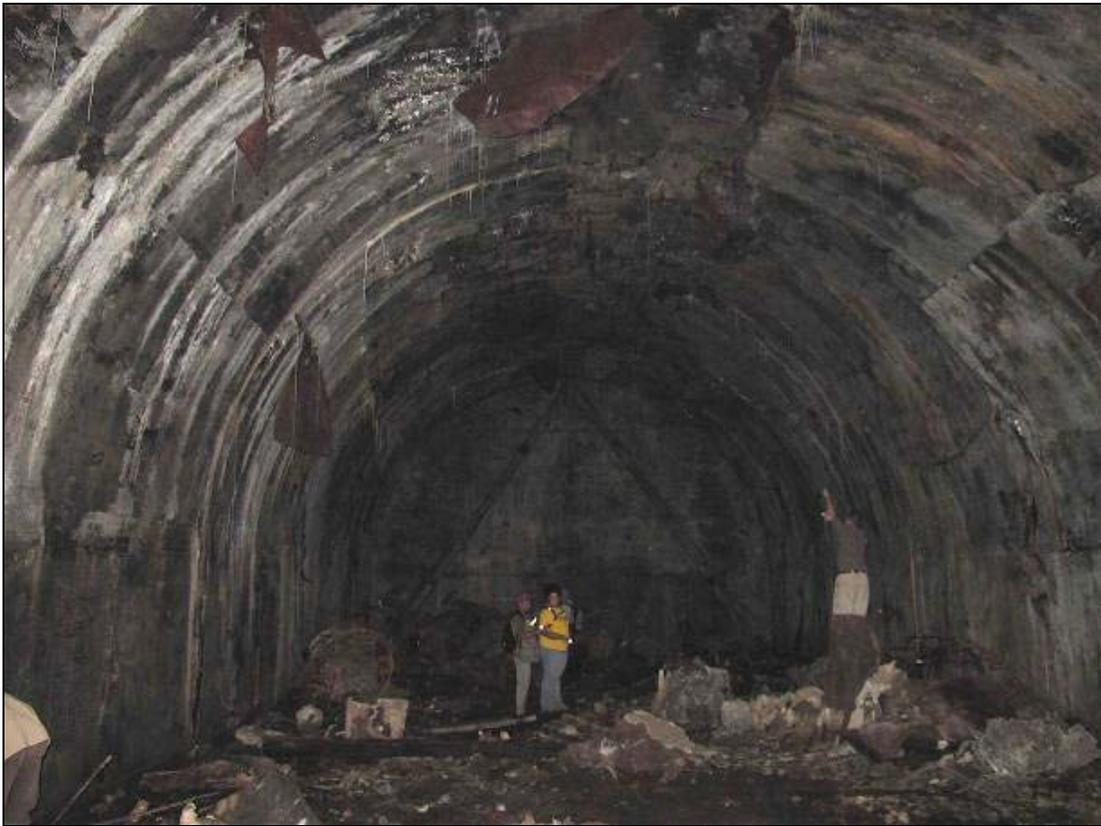
**Figure 6.21** Interior of the concrete lined Japanese storage cave at site AB145.
